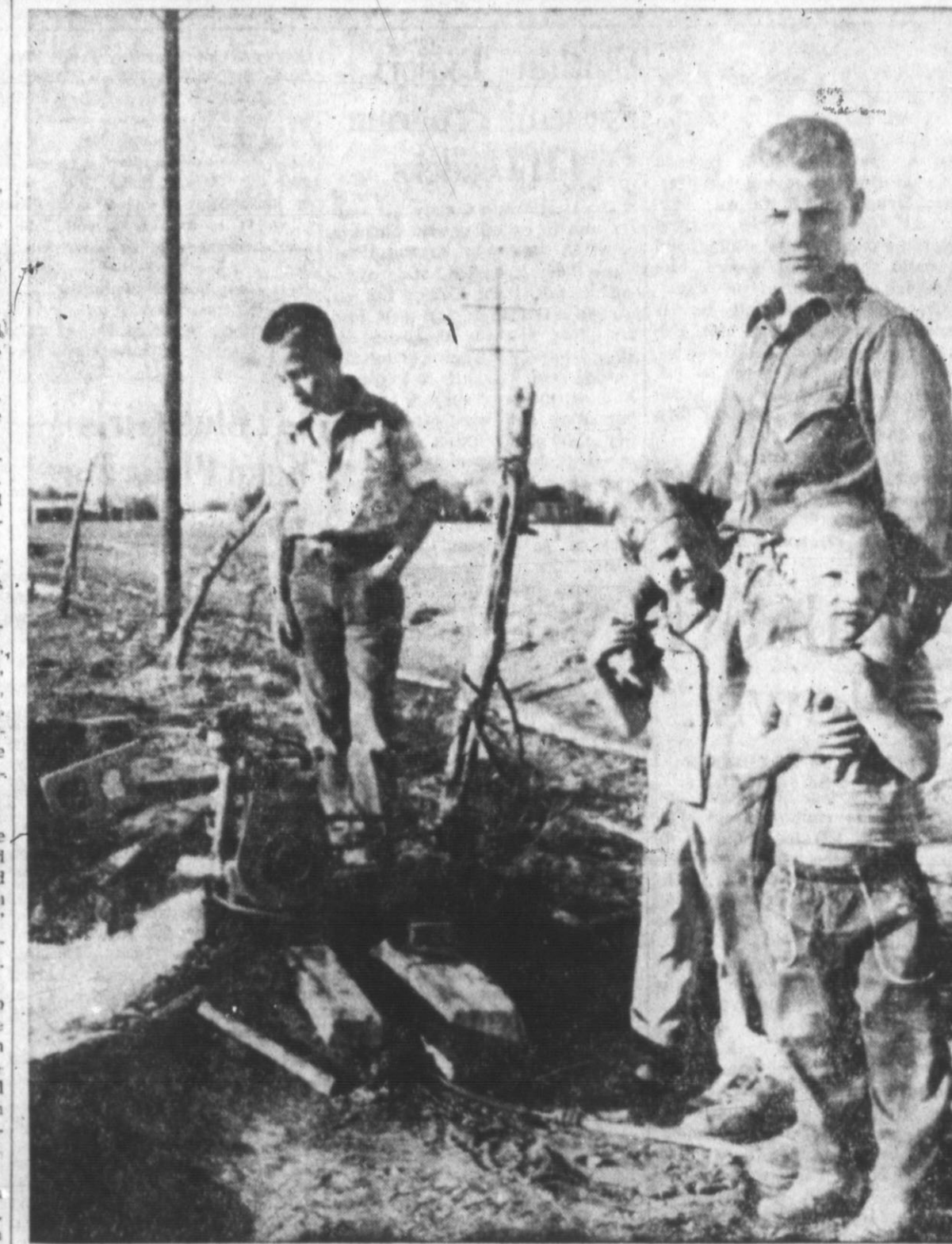
FRANK SCOTT watches a full four inch pipe of water flow from the handy little pumping system made by his father Jesse Scott who "figured out" the arrangement to utilize water flowing from onions and other crops up the ditch from their home on Country Lane southeast of Hereford. Shown with Frank are Sally and Terry shyly clinging to big brother Don. (Staff Photo)
