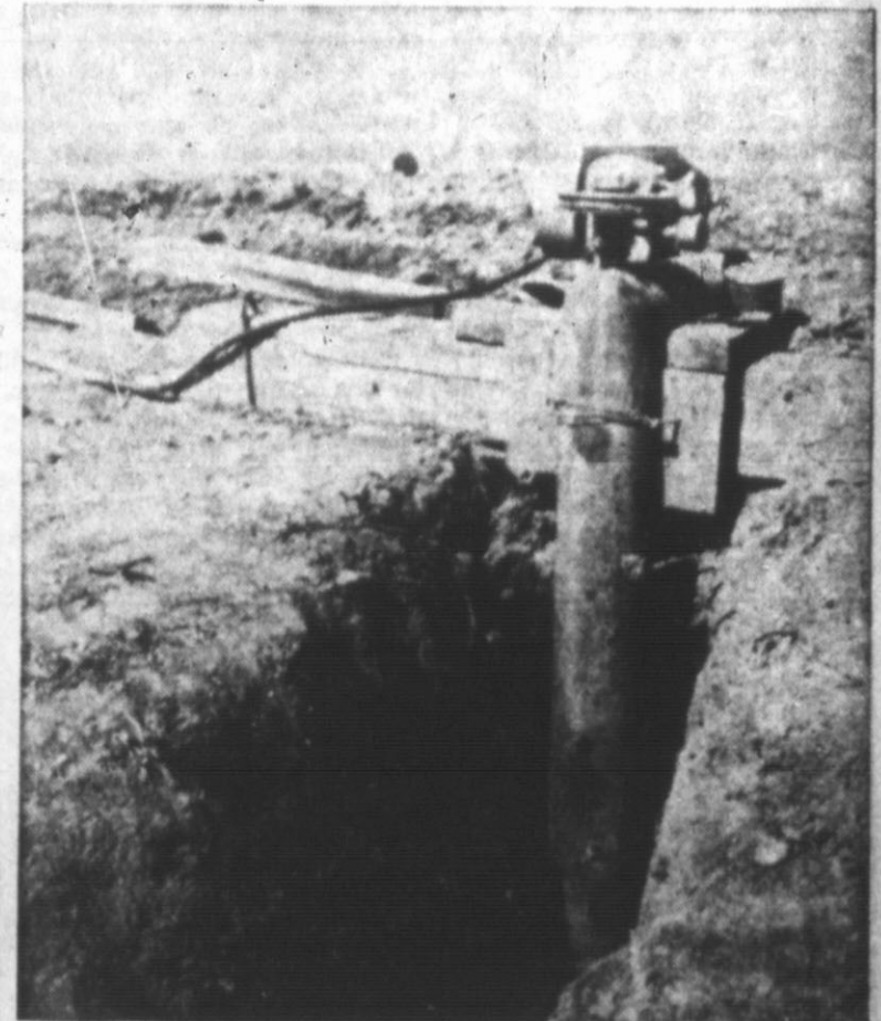
A CLOSE-UP of the pump and motor which furnishes the power to rotate the auger from an old combine placed inside a four inch pipe and connected to a pulley operated by one and a half horse power motor which uses butane for fuel is shown. The whole set-up is portable and is easily moved to different locations along the ditch for convenience. (Staff Photo)
