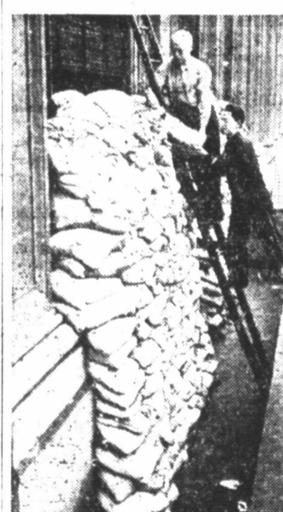
Completing the job of placing sandbags outside the office windows of Hotel Bossert in Brooklyn. The barriers were installed so the hotel organization could keep functioning in case of an air raid.
