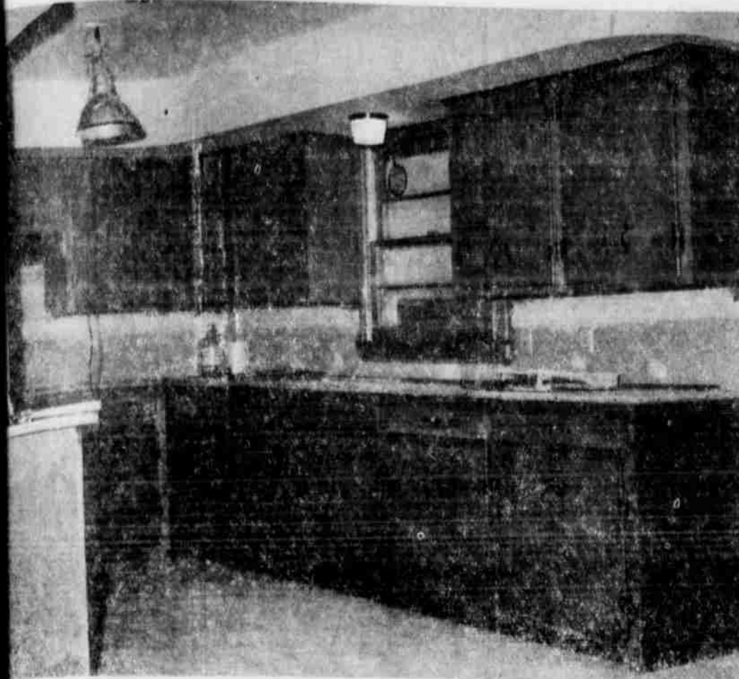
KITCHEN —This kitchen in the O. B. Graham Jr. home at 117 East 18th Street is paneled and features a copper stove, antique maple finish cabinets and copper hardware. Builder was Hall Construction Co. of Lubbock. (STAFF PHOTO)
