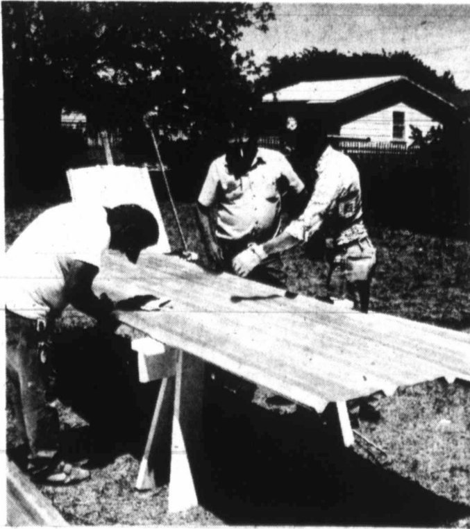
Ken Whitzel and company cutting tin for a roof.
