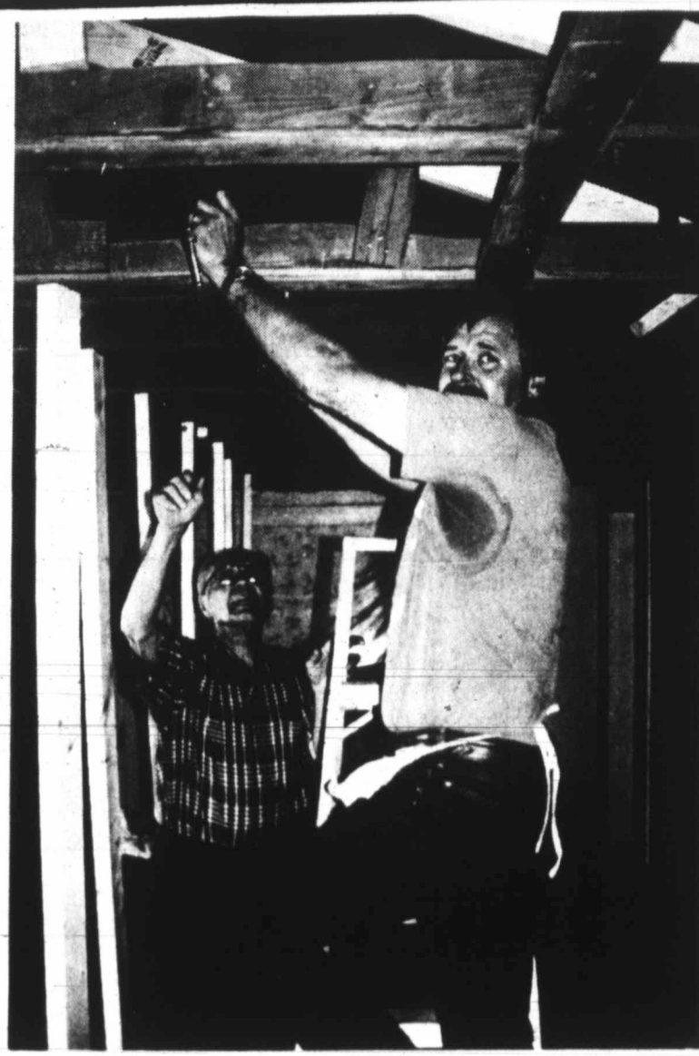
Ron Goebel and George Witten putting up a ceiling.
