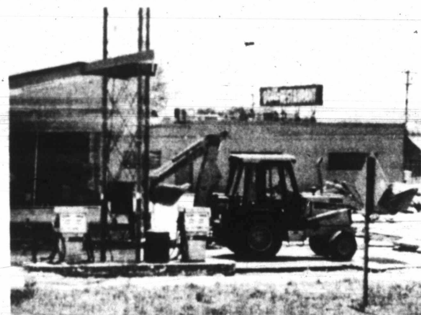
NEW BUSINESS: McCormick Marketing of Snyder has begun construction on a new convenience center to be located at the intersection of Hwy. 208 N. and I-20, where the existing Willis Taylor Phillips 66 station has been in operation for years. The center will also contain a Burger King and Blue Bell Ice Cream store. Opening date is set for August 1.
