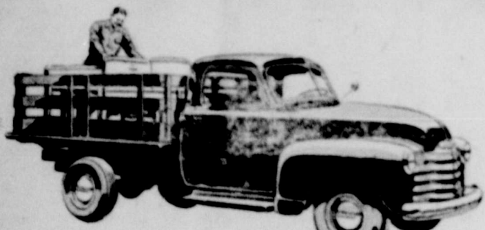
MEDIUM-DUTY DE LUXE STAKE* Model 3600—125 1/2 inch wheelbase, Maximum G.V.W. 5,800 lb. Other models available on 151 inch wheelbase and 16,000 lb. G.V.W.
