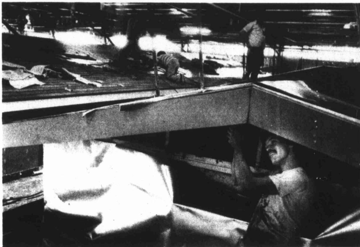
INSULATION — Workers at Cameo Energy Homes work on insulation and roofing of two manufactured homes at the Cameo production site. John Beddow,
