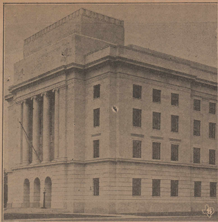
Here is a Federal Building unlike any other in the United States. It has just been completed at Tezakama. The state line between Texas and Arkansas runs exactly through the center of the building. The postoffice occupies the first floor and basement. Above the first floor the structure is virtually two separate buildings, divided by a solid wall. The structure costs a million dollars complete.
