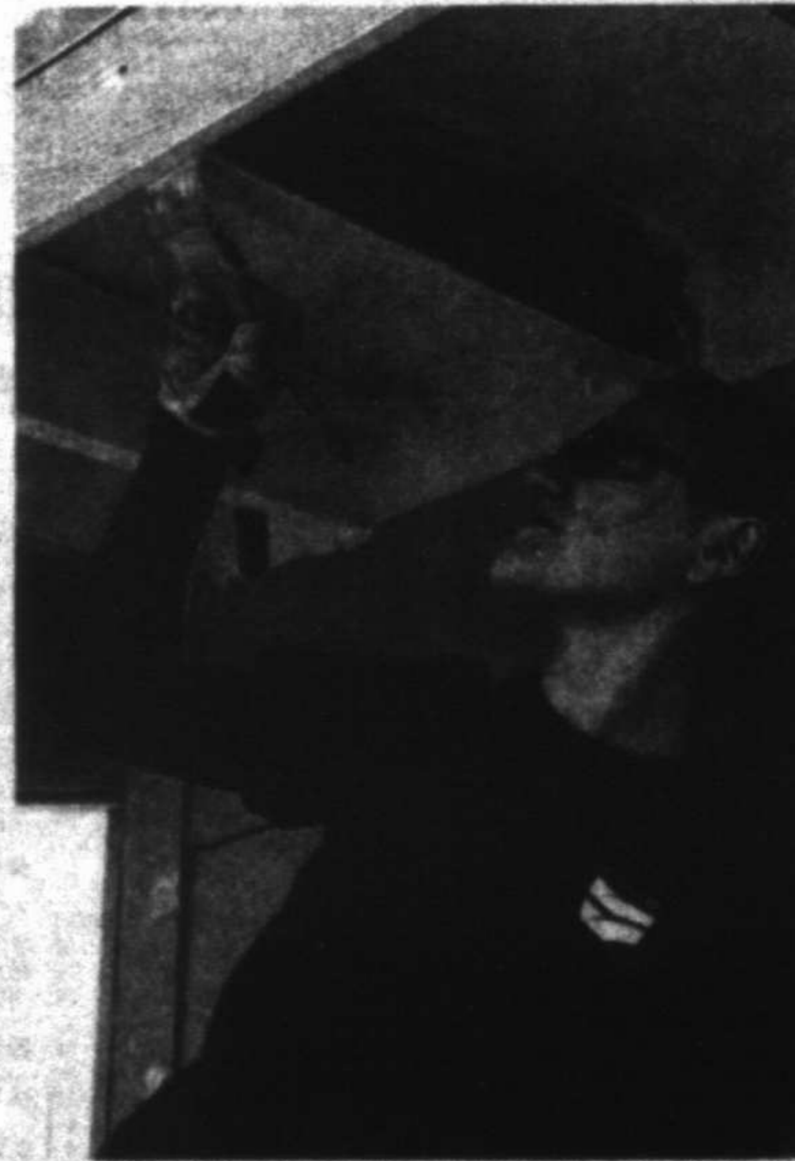
Anna Letyshova, with Chevron, paints the roof eaves Friday to a home on East California as she and others with Chevron work to repair the house as part of Christmas in Action.
