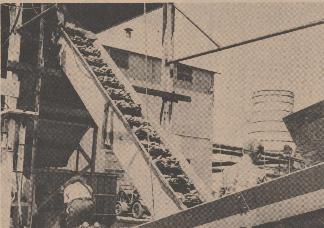
PRACTICALLY PICKLES -- "Heart of the grading operation" is this large conveyor which lifts cucumbers to the sorting phase of the operation. In the foreground can be seen the conveyor which removes "culls" - oversized or malformed cucumbers.
