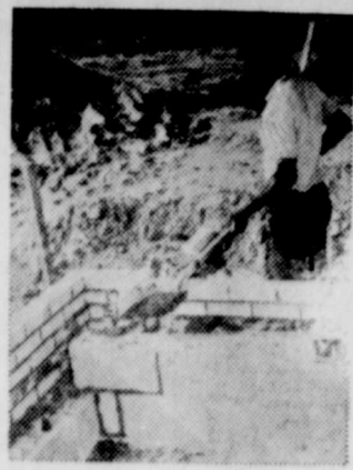
WORKER FILLS the hollow cores of wall blocks with sand to provide added shielding mass against radiation—one of several techniques used to build low-cost fallout protection into a new church at McLean, Va.
