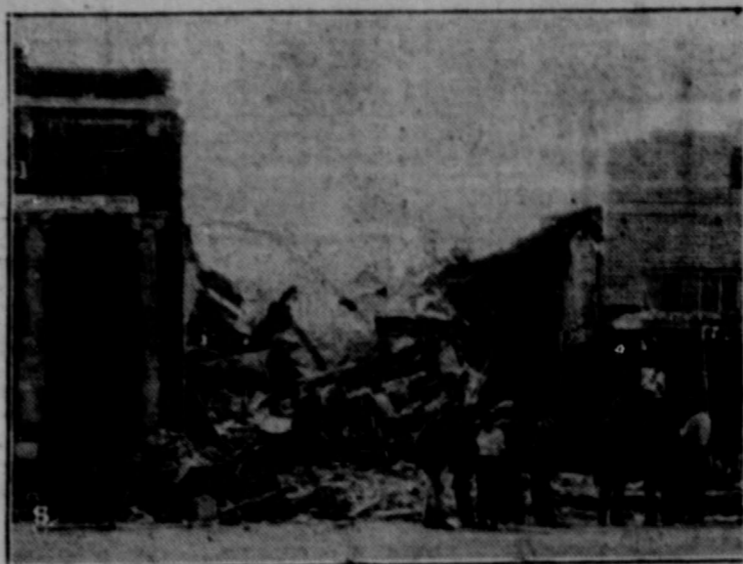
Here is the scene of the downtown gas explosion at Panhandle, Texas, which resulted in injury to four people and $50,000 damage. The blast occurred when W. H. Rogers, grocer, struck a match to look for a gas leak. Rogers, J. L. Raines, Roscoe Vance, Ed Baker, and his son, Enzo Baker, were all injured, and three buildings were damaged, one being completely demolished.
