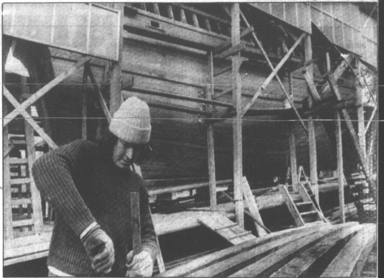
WORKING WITH GODSPEED —Kenny Cole Jr. works on the treated deck beams for the rebuilt 17th century ship Godspeed at the Yorktown, Va., Boat Shop. The ship
