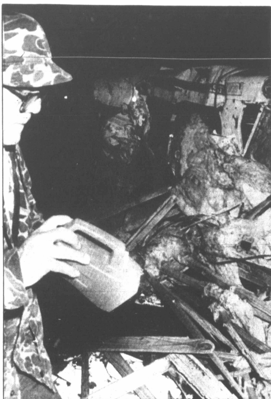
SEARCH—A rescue worker searches the wreckage of a house in Fisher, Ark., after a tornado ripped through the area, killing three persons and littering the countryside with debris Thursday night. (AP Laserphoto)
