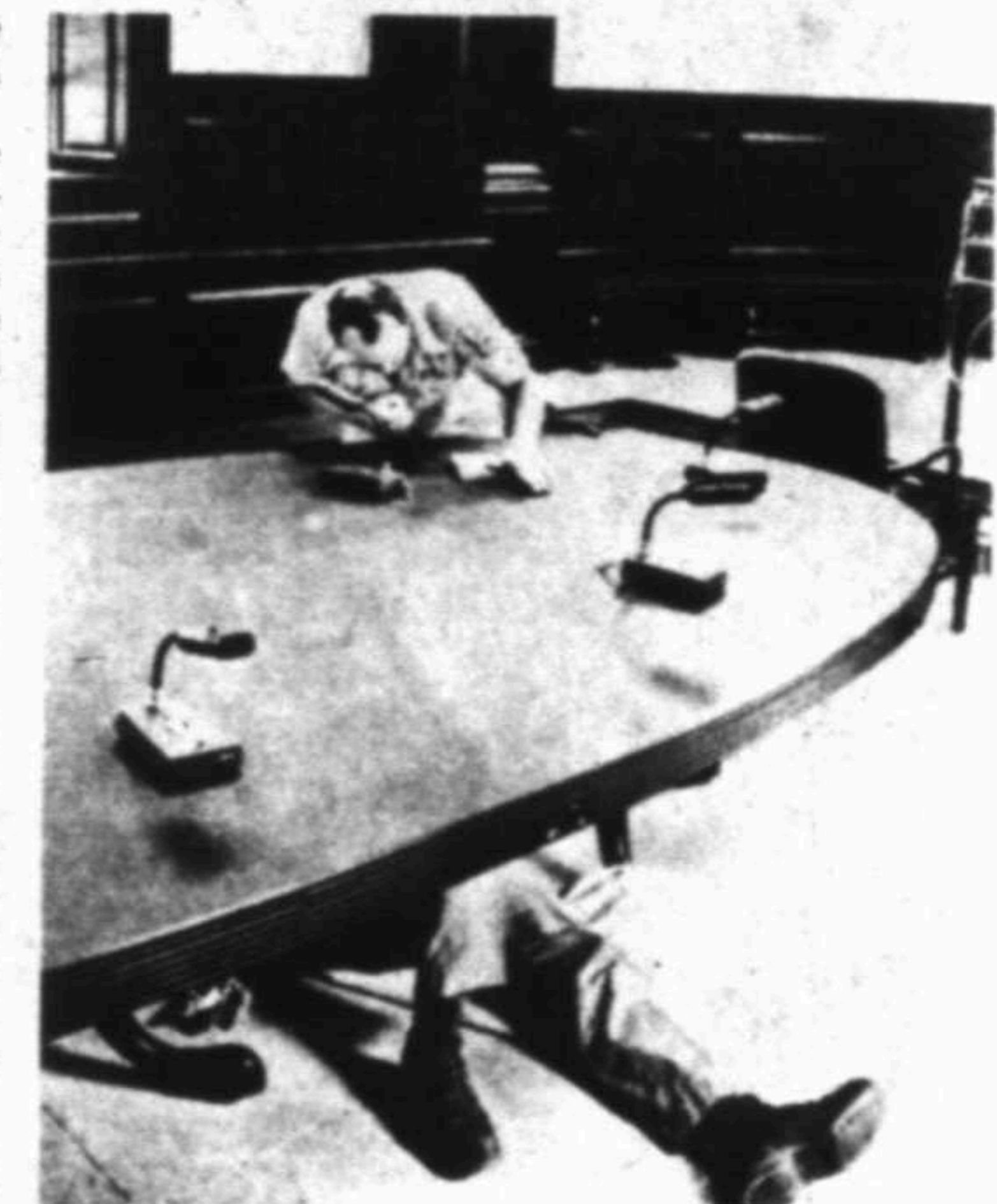
Electricians wire a table in the House of Burgesses, where heads of government from seven nations and the European Common Market will gather.
