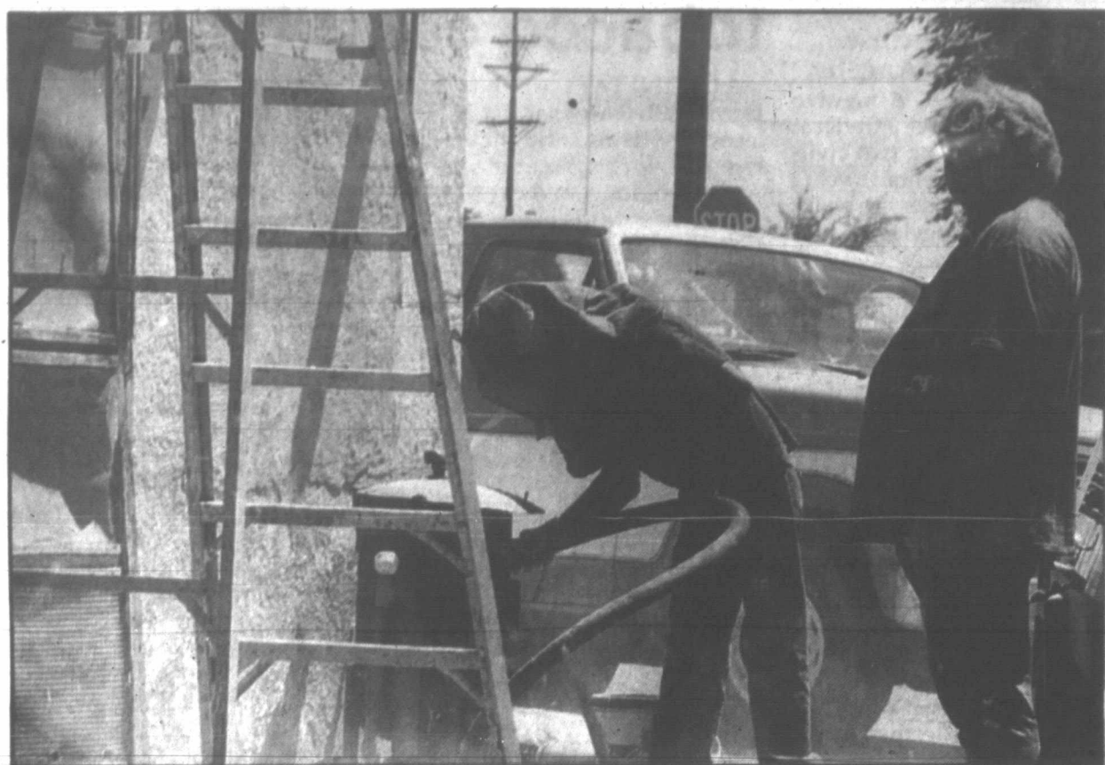
(Pampa News photo by Danny Cowan) Downtown drivers passing by the intersection of Somerville and Foster earlier this week may have thought there was a dust storm brewing. Instead, the cloud came from sandblasting efforts by Leonard Provence, left, with Billy Swanson looking on, as they work on renovation efforts for a building at the intersection.
