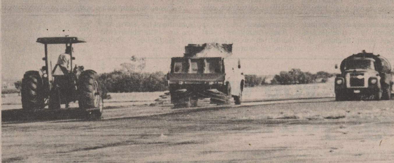
RUNWAY WORK — A seal coating project is now underway at the Scurry County Airport involving both Scurry County and City of Snyder personnel. The work
