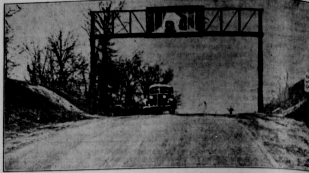
TRAFFICSCOPE WARNS ONCOMING MOTORISTS OF APPROACHING CARS
