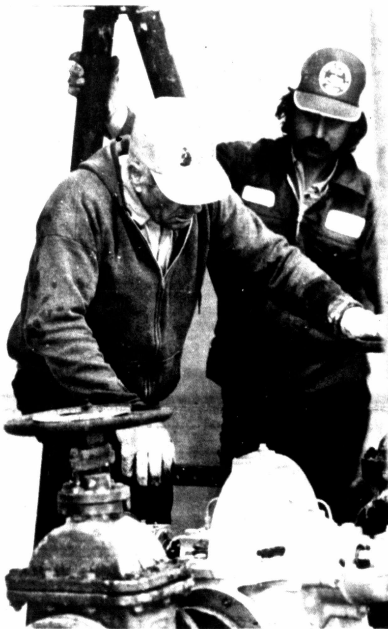
QUICK REPAIR — Kenneth Rinehart and Alvin Dodson, city employees, are pictured changing out a coupling on a water pump this morning near the Hwy. 84 bypass. The problem was not expected to effect water service in the community. (SDN Staff Photo)
