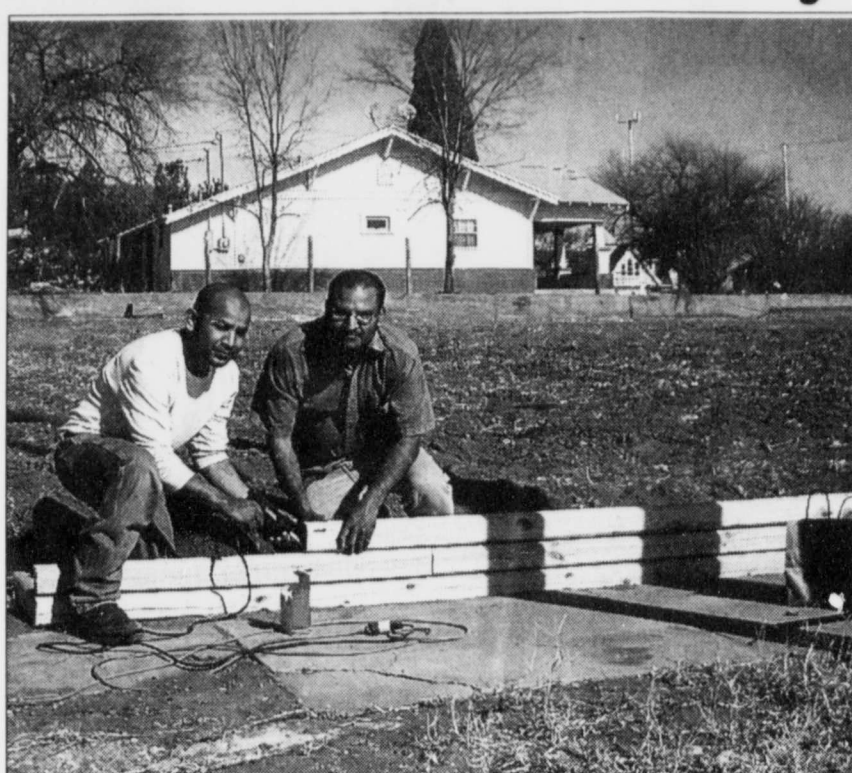
TWO VOLUNTEERS Tim Arocha and Rusty Medrano built the retaining wall at the future site of the KCCB sponsored Community Gardens located at 3rd and Hickory Streets. Photo courtesy of Julie Erwin.
