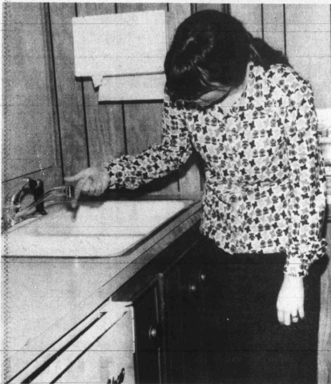
A LITTLE DRIP, A WHOLE LOT OF WASTE — Sharon Hooper investigates a faucet for a leak. If a steady drip occurs, thousands of gallons of water can be wasted in a month's time, resulting in unnecessary water bills. A gasket which often can be installed by the householder can usually solve the problem.
