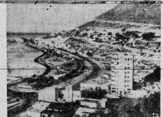
CITY HIT BY QUAKES AND TIDAL WAVE—This is an aerial view of the shoreline of Agadir, Moroccan city of 40,000 on the Atlantic coast which was shattered by two extensive earthquakes and a tidal wave. (AP Wirephoto)
