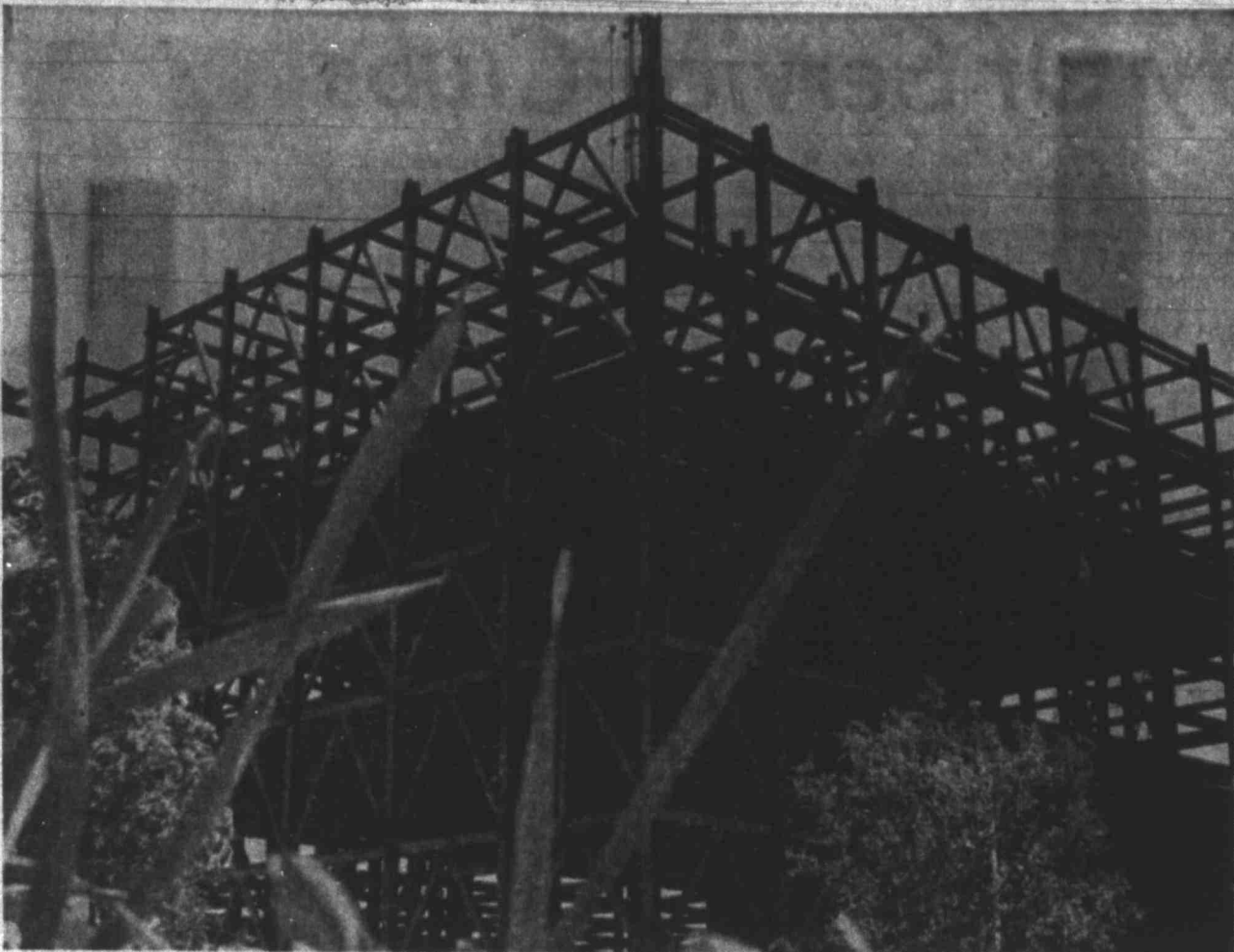
GROWING WITH MIDLAND — Southwestern Bell's new seven-story, $17-million electronic switching center is beginning to take shape.
