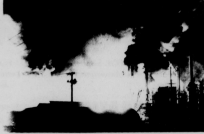
MINERAL WELLS EXPLOSIONS AND FIRES DESTROY GAS AND PIPELINE FACILITIES plus nearby property. Fortunately, it happened at 1:58 A.M. with only one slight injury reported at the time.
