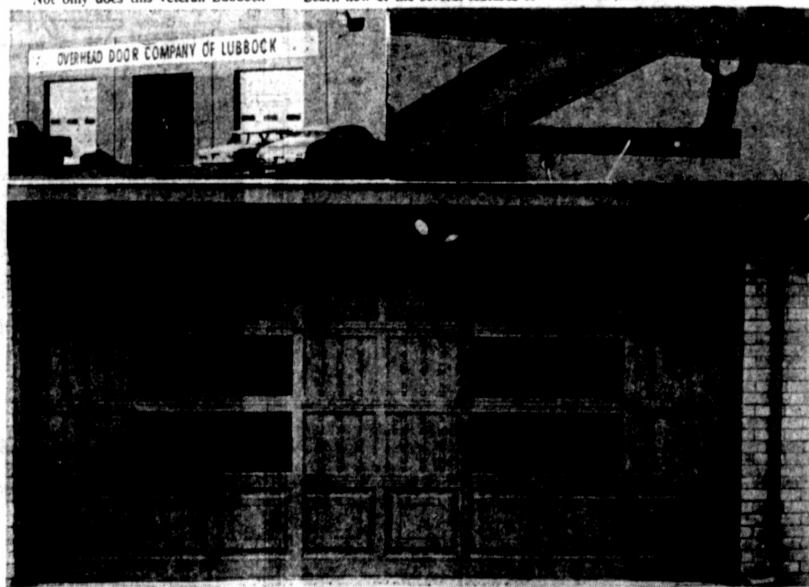
REALISTICALLY A CONVENIENCE, SAFETY FACTOR — Shown is a Lubbock installation of an overhead automatic door from Overhead Door Co., 50th Street at Frankford Avenue, with (upper right) the popular automatic opener that can be a lift in your own situation, whether for a new or existing home. General Aluminum windows also are distributed by the Lubbock firm.
