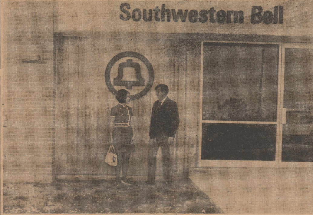
Mayor Delmar R. Hiller and Miss Virginia Hill, manager for Southwestern Bell, are shown in front of the newly constructed central office of the Telephone Company at 115 North Pearl Street.
