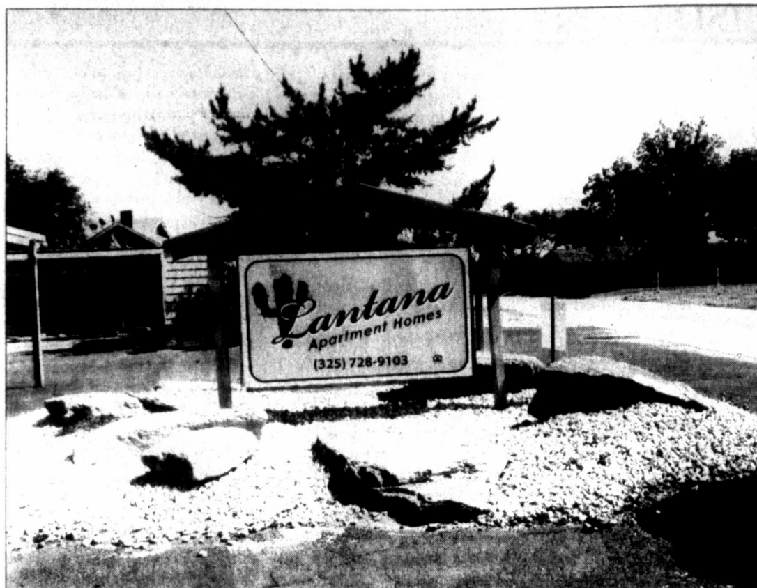
NOW TAKING APPLICATIONS – Apartments in the Lantana Apartment Homes complex have been modernized, updated and completely renovated. Manager Judy Bartels of the complex located on 10th Street is taking applications for prospective tenants.
