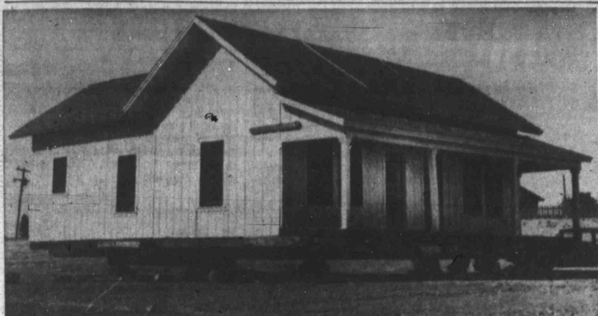
OLD BUILDING WAS MOVED IN... but it will be replaced by entirely new structure
