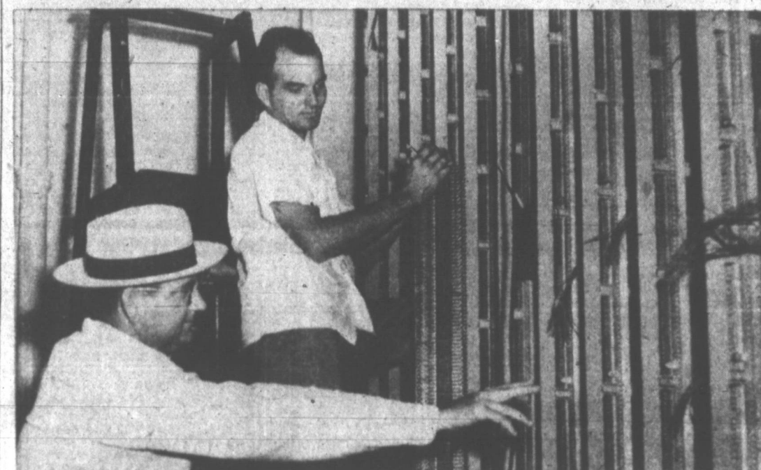
MAIN CABLES FOR DIAL SYSTEM in Pampa are being installed at the local telephone company. To be run from Amarillo offices, the cables, totalling 7,500 pair terminate in the upstairs part of the new local structure. Above are J. D. Miller, left, division cable splicer foreman, and a member of his crew, Max Florence.
