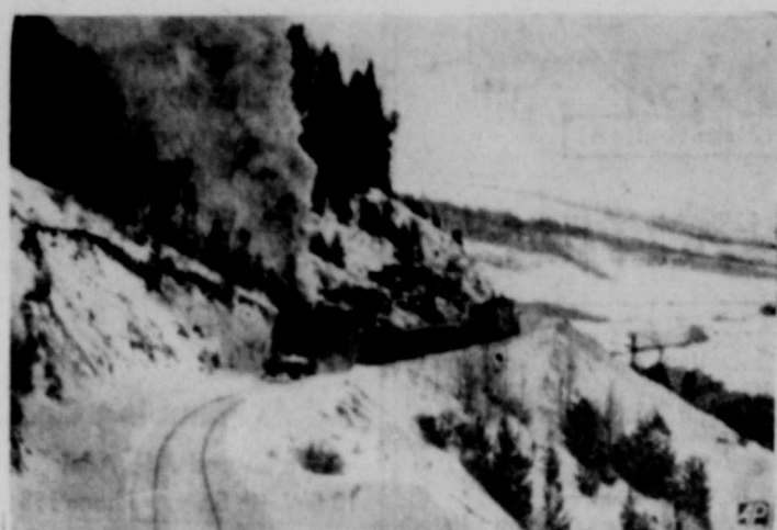
LOTS OF CURVES—The Laramie, North Park and Western railroad claims a place among the most winding railways in the world. It has fifty-seven 12 degree curves in its 111-mile long main line. Sometimes even the conductor gets dizzy on the run, they say.
