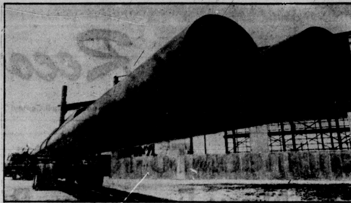
DON'T SHOOT —Twin barrels of a huge shotgun? No, just long steel plate tubes, three feet in diameter. The tubes are part of 40,335 linear feet of piling produced for a port development project along the Baton Rouge, La., waterfront.
