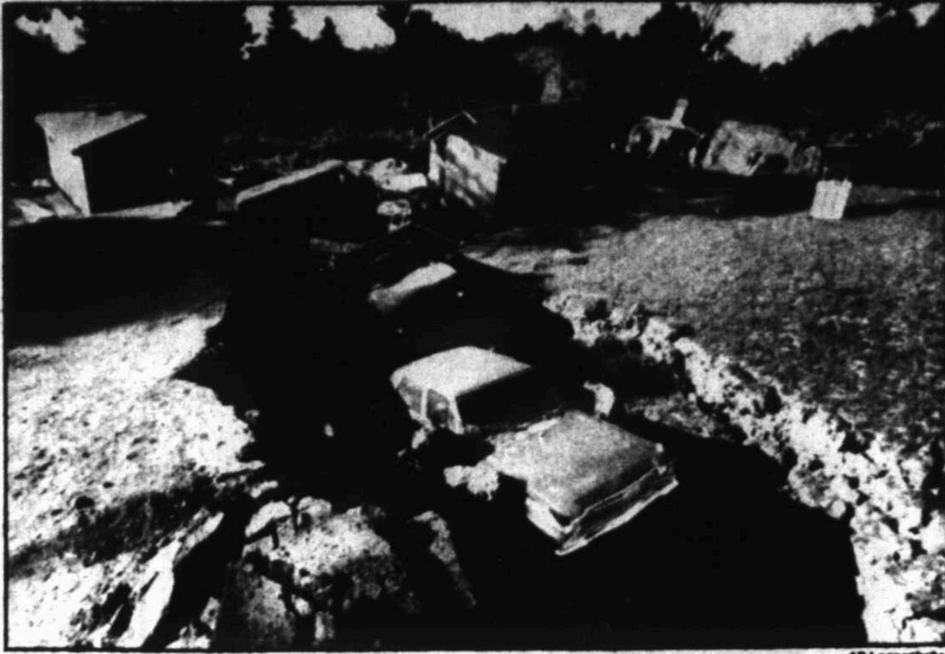
A freak landslide in Gorham, Maine on Wednesday demolished a newly finished house and four vehicles while eight people narrowly escaped injury. The 500-ft. wide slide created nearly a 20-ft. vertical drop where the cars and house were located.
