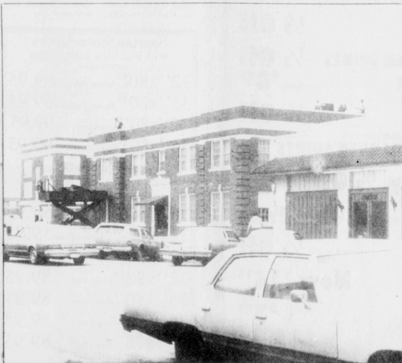
CREWS FROM Lydick & Hooks of Abilene work on the city hall roof Tuesday morning. Light showers cut their work short just a few minutes later. Cold weather hampered the company's work in Colorado City for much of December.
