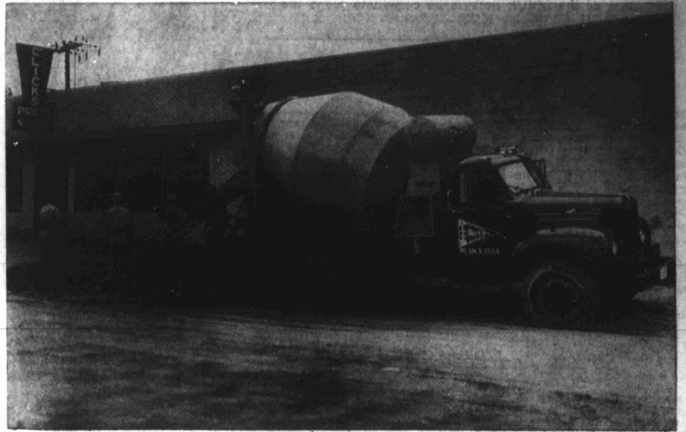
Shown is one of our brand new Mack Trucks unloading cement on the job. This truck has a capacity for mixing and delivering 8 cubic yards at a time. We have sizes for all jobs.
