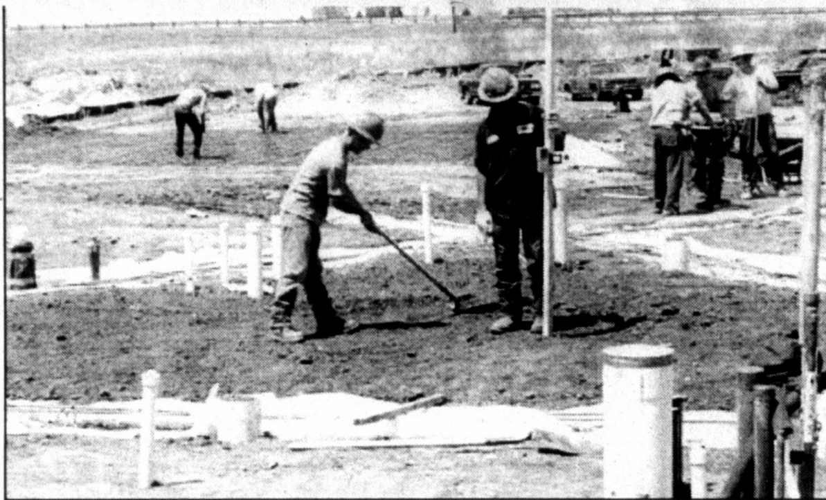
HOSPITAL CONSTRUCTION WORKMEN readied ground for insect control spraying preparatory to pouring concrete. Steel erecting has passed the halfway point at the Rogers Road and South Interstate 20 site.
