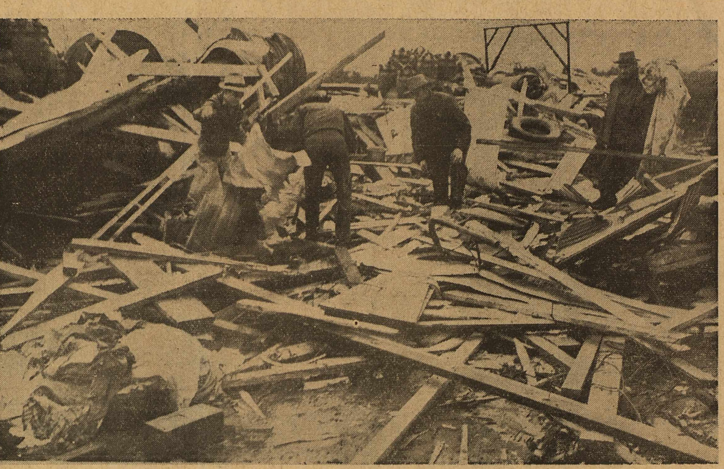
Heavy pumps managed to withstand the battering of the tornado that struck in Rodessa, but all around can be seen what was left of "supply company row," in the center of the damaged area, with oil field roustabouts digging through the tangled mass. Twenty-two persons were killed and 50 or more injured in the worst disaster that has ever struck the oil town. Property damage was estimated at $500,000.
