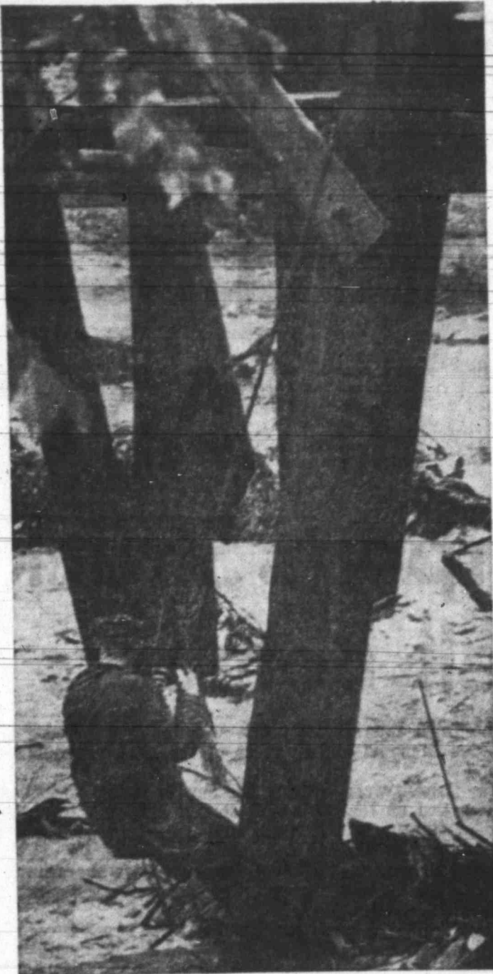
Trestle In Trouble
