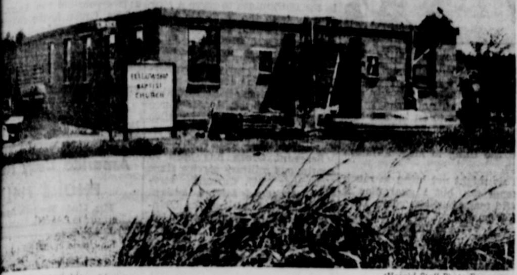
COMPLETION —The new building of the Fellowship Baptist church, S. Ash and 6th avenue, is nearing completion. The concrete block walls of the structure have been erected and workmen are on the roof now.
