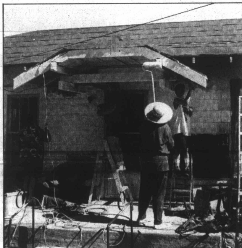
REFURBISHMENTS abounded Saturday at the 236 Central St. home of Pablo Martinez, where members of the First United Methodist Church led the Christmas in April project to repaint and re-roof Martinez' home and put new electrical wiring in it.
