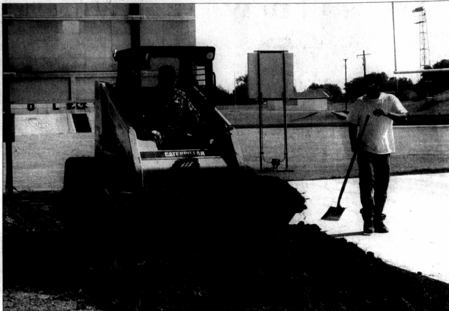
BEGINNING THE FINAL PHASE - Work continues on the Colorado High School track, as Isidro Fraere (left) and Simon Favila (right) from Texas Sports Builders backfill curbs and wait for the base rock to dry after recent rains. Workers will begin pouring the asphalt on Monday, according to Robert Wheeler, of Texas Sports Builders.
