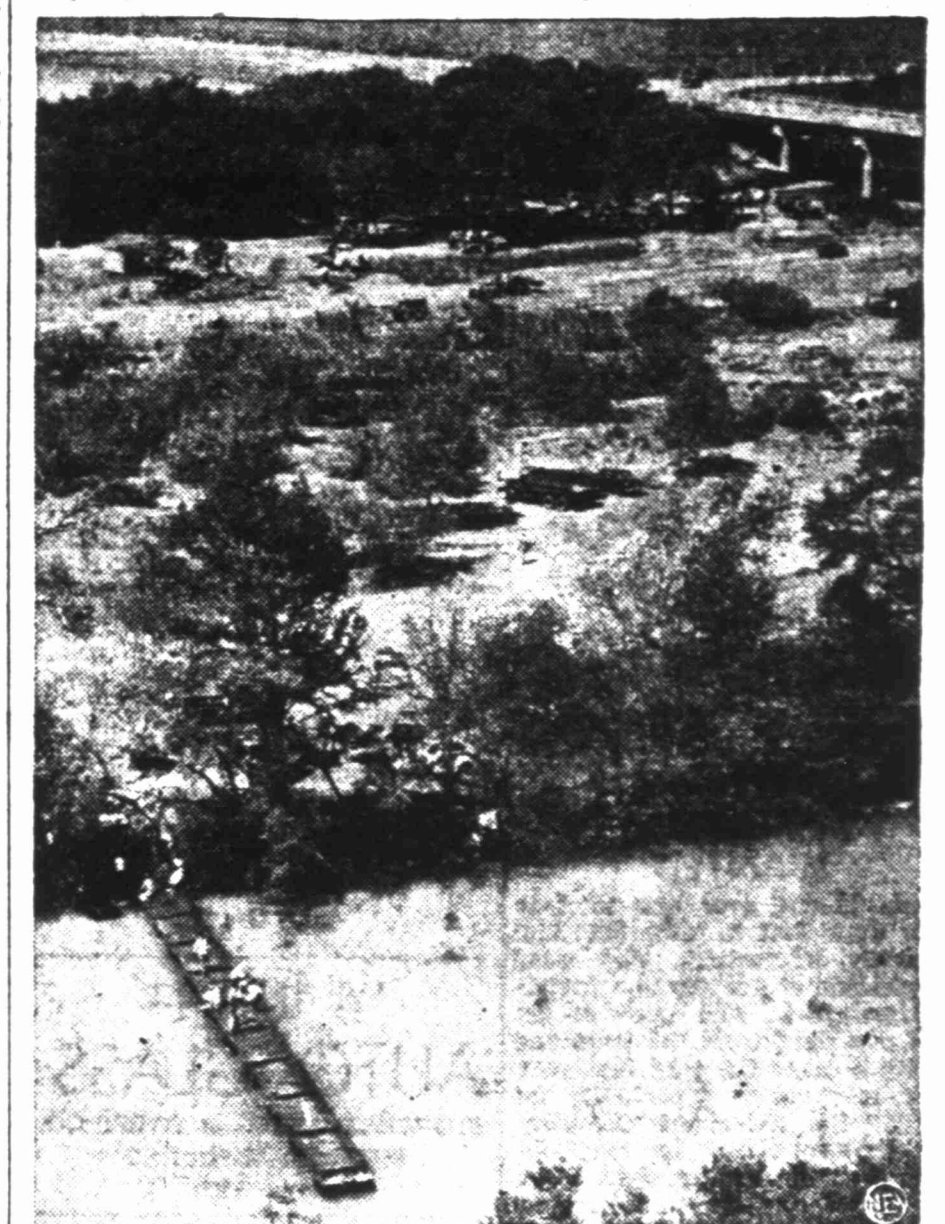
Kerrville's "Build a Park in A Day" project looked like this from the air as half the town pitched in. Pontoon bridge (foreground) is the same one in the other photo.
