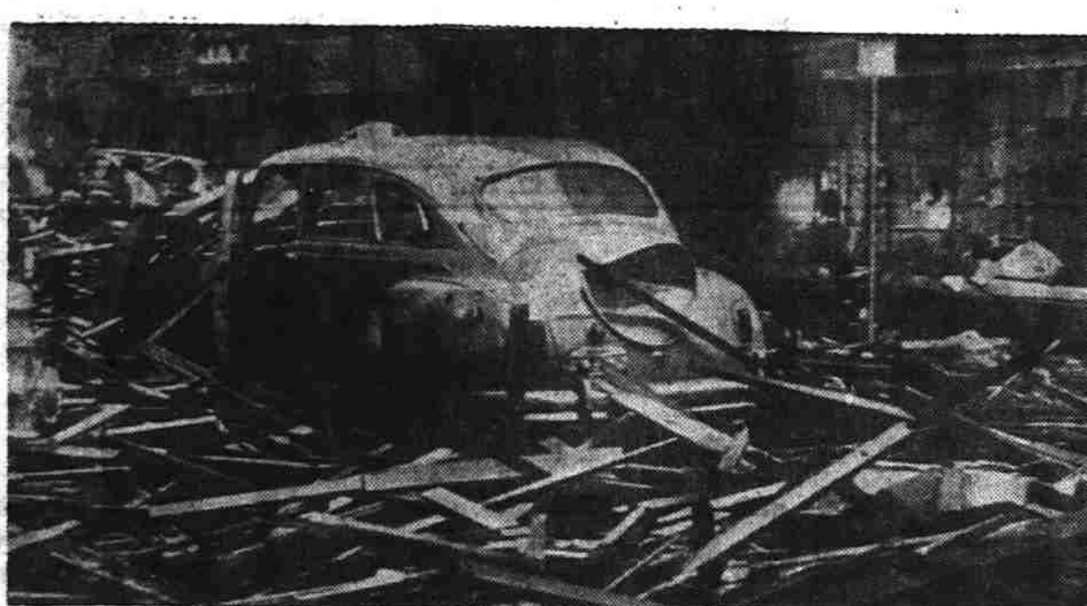
HURRICANE DAMAGE — Debris litters this downtown street in New Orleans after a hurricane ripped through the city. The rubble was formerly a house on top of a tall building and housed a cooling system. (AP Wirephoto)
