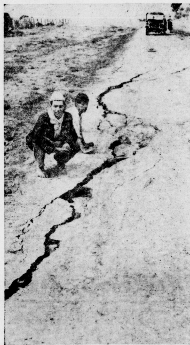
A GRIM REMINDER —Long, deep cracks in the highway near San Jose, Costa Rica, recall to Bernardo Amador Chando, left, and his brother, the violent earthquake that struck the area after Christmas. Bernardo's wife and six children perished in a mile-wide landslide that engulfed his home while he was at work a short distance from it.
