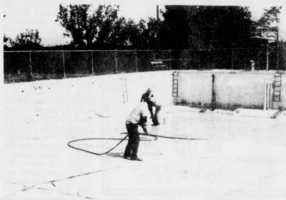
GETTING IT READY - City workers are hard at work getting the city swimming pool ready to open. The pool might possibly be open by this weekend. Supervisors for the pool this year will be Tom Ramsey and Mark Merrell.
