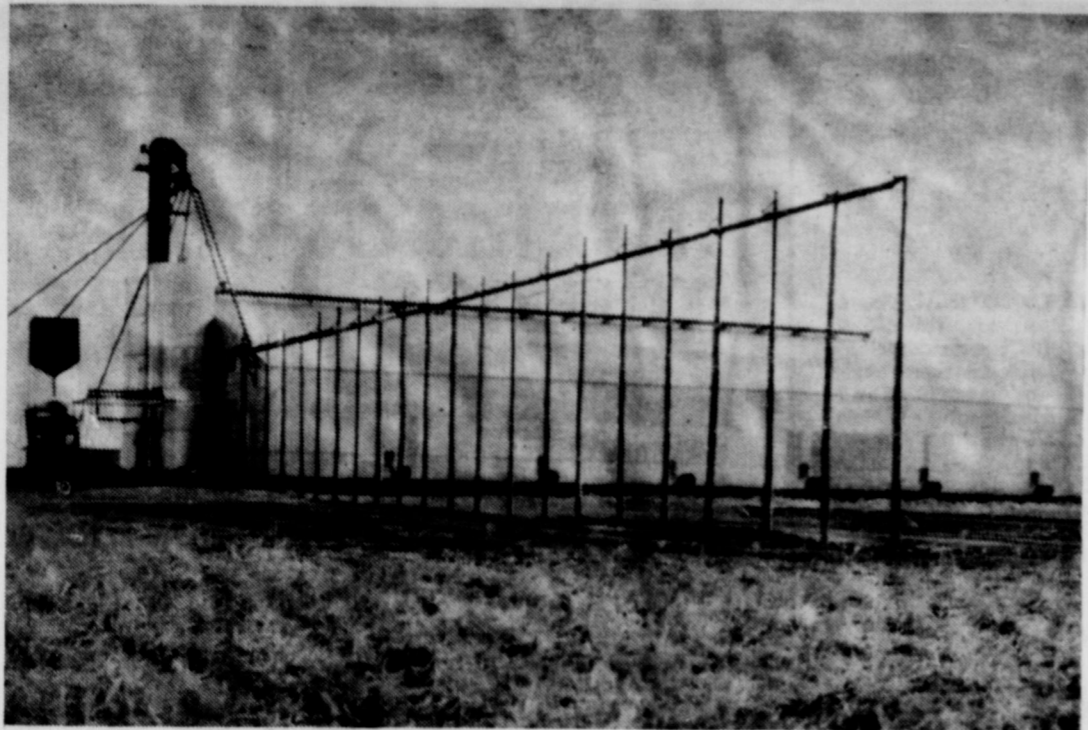
PAR-LAM STORAGE WAREHOUSE IN LAZBUDDIE
