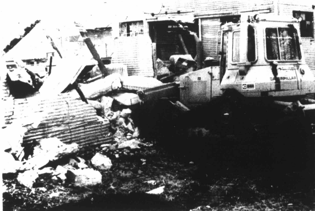
DEMOLITION CONTINUES—City crews tackled the old gin on West Highway 80 this week, knocking down the still sturdy concrete walls which are re-enforced by 4-inch pipe. More than 20 substandard structures have been razed by the City and others will soon be targeted.
