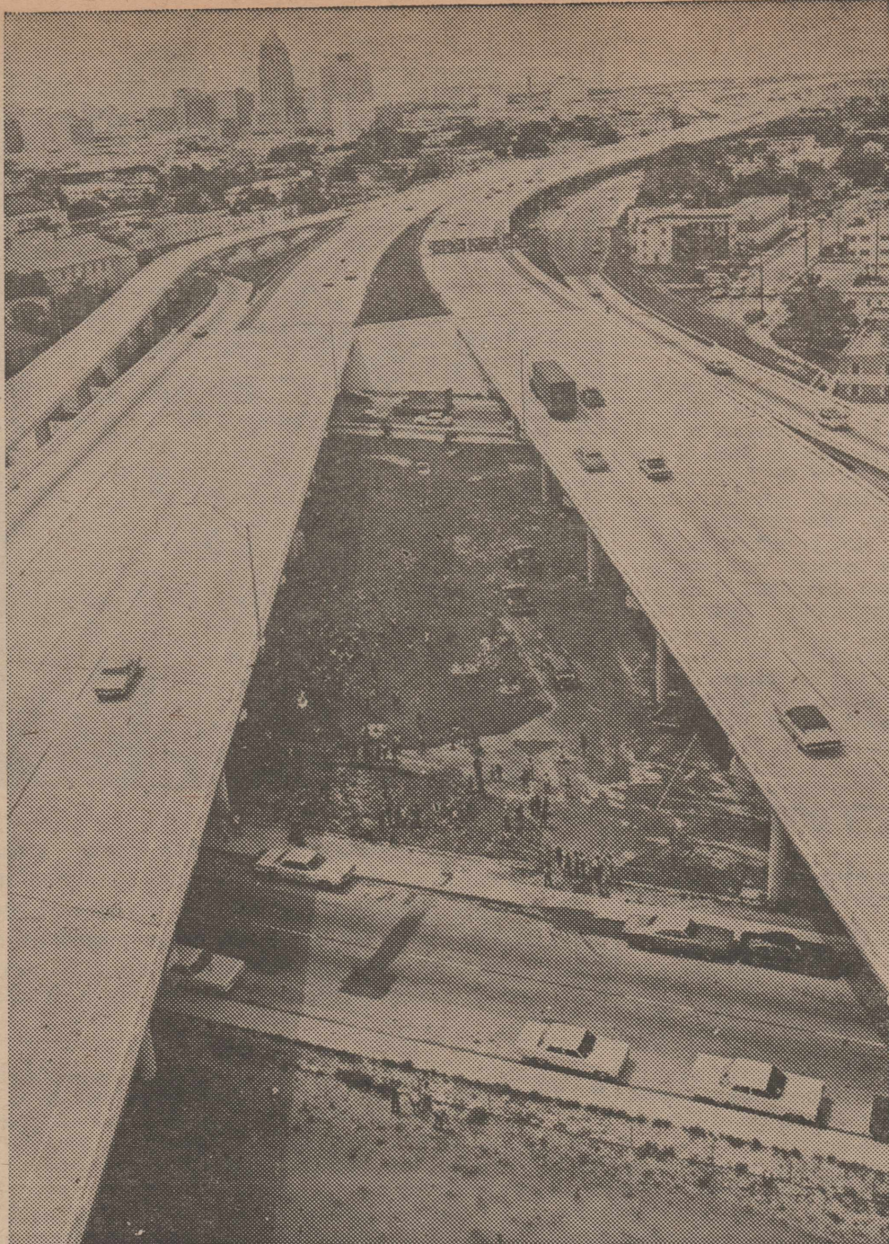
UNDERNEATH IT ALL, children play. While automobiles hurry along this expressway toward downtown Miami, Fla., youngsters enjoy the new M. Athalie Range Park which has been created in the valuable-but-unused space beneath highway.
