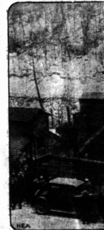
Nineteen miners were killed in a blast several thousand feet down in the Junction Coal and Coke Company shaft at Farmington, W. Va. This hoisting shaft is directly above the spot where the explosion happened.
