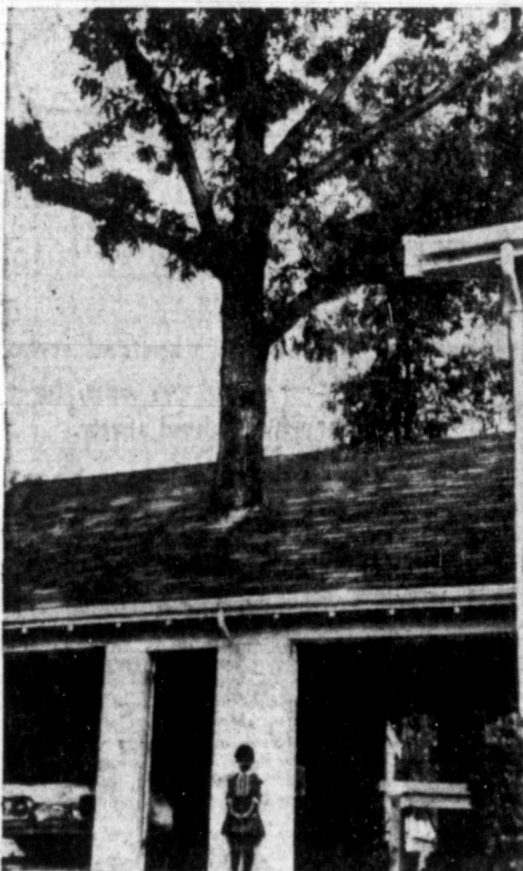
SPARE THAT TREE —This oak tree in North Attleboro, Mass., was so much a part of the Moulton family, they couldn't bear to part with it. When the Moultons needed an extra garage, they built the extension around the tree, which was abutting the outer wall of the first garage. Sighing with relief, the tree is flashed to bend easily in the wind.
