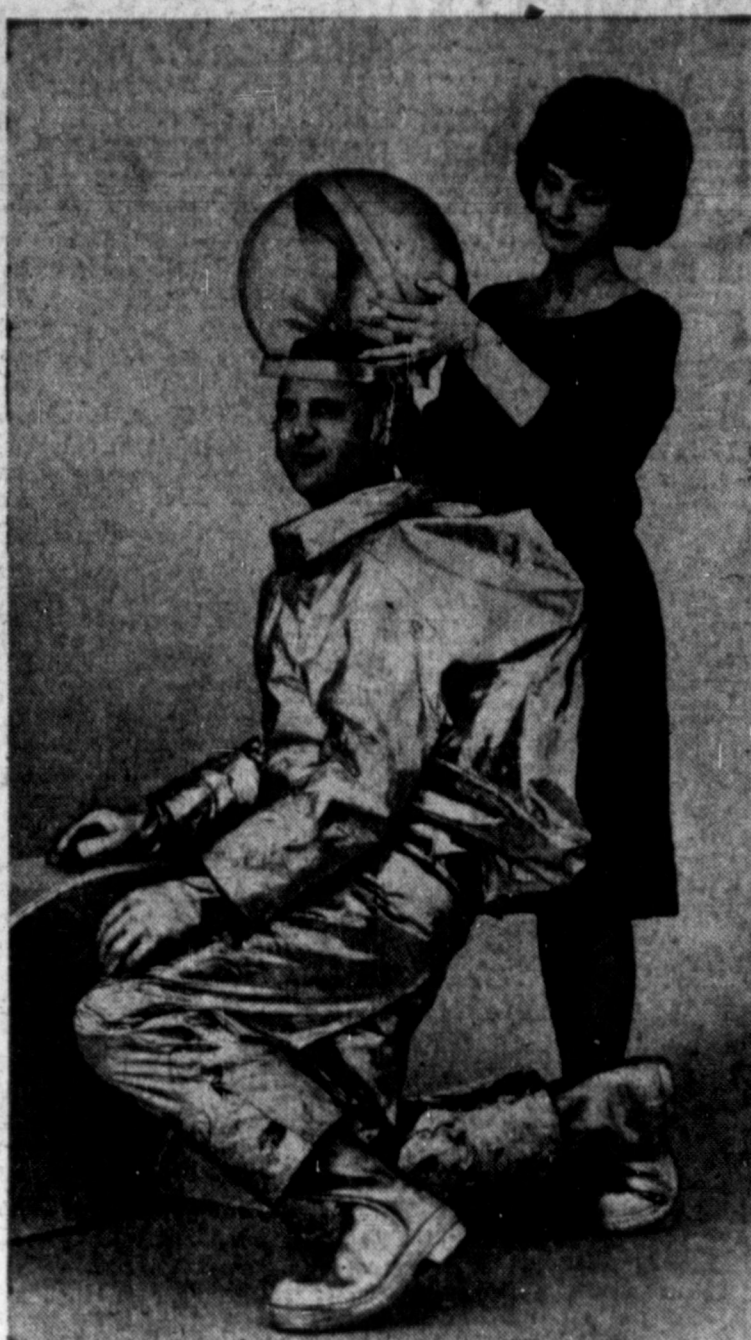
GOLD SUIT FOR SPACE AGE WORKERS —Paulette Hale helps engineer William Phillips with the plastic helmet which completes this 24-karat gold outfit for missilemen. The Armalon fabric is surfaced with pure gold and gives protection from flash temperatures up to 3,000 degrees F.
