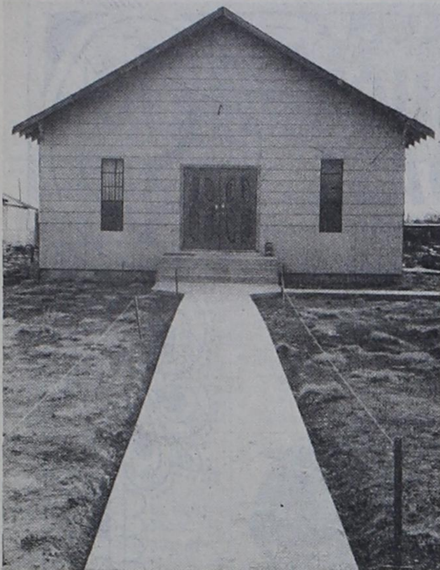
A NEW LOCATION —La Asamblea Christiana congregation in Dimmitt has moved its meeting house to this location at 400 NE Fifth Street. Remodeling, new windows and siding, new doors, and new carpet and paneling were all added to the building, which will also have a new 30-foot extension built on for classrooms and possibly a kitchen, according to pastor Rev. Ruben Velasquez. The approximately 100 members of the congregation have done much of the work themselves, and hope to have it all completed before winter. The building used to be located on Southwest Fifth Street in Dimmitt.
