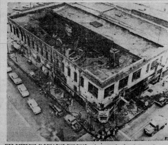
FIRE DESTROYS BLOCK-LONG BUILDING —A spectacular fire that roared out of control for several hours in downtown Dallas left this block-long building with only part of the roof and walls remaining. Six firemen were injured when the ceiling collapsed on them and 14 others were treated at the scene for smoke inhalation. Damage was estimated at $150,000. (AP Wirephoto)
