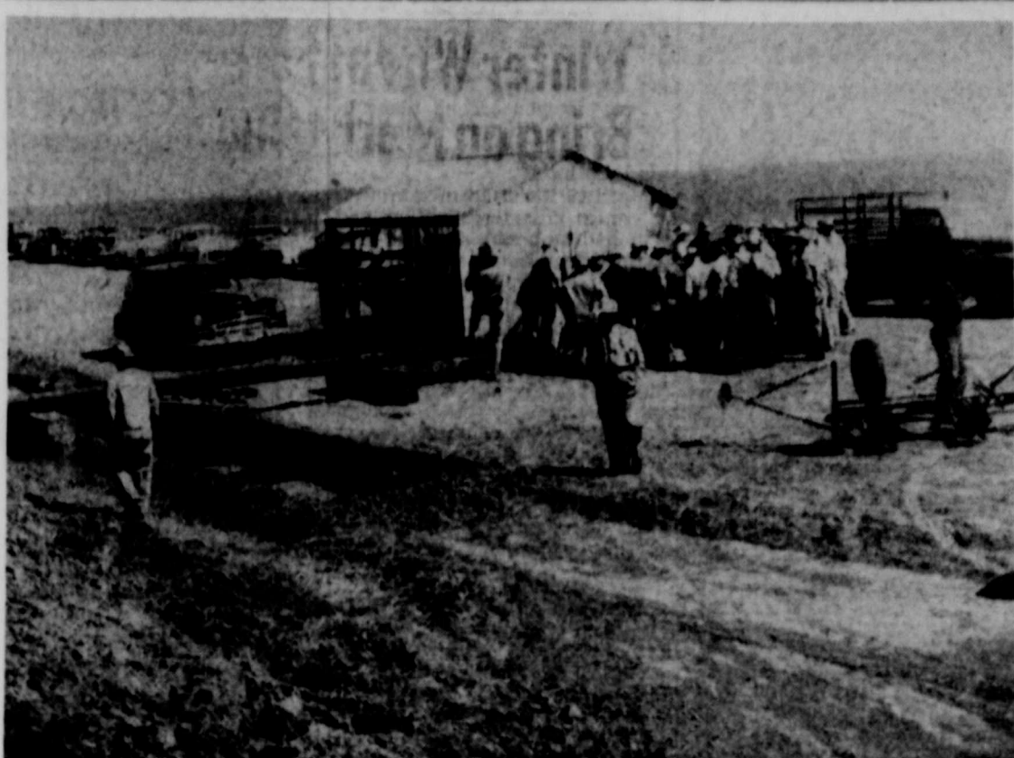
AT HAWK WELL —Visitors look over the pump and well at the Harlan Hawk farm near Farnsworth on the Tuesday irrigation tour. This well, powered by a motor operated on natural gas, delivered 1,010 gallons per minute in a test run made for four visitors.
